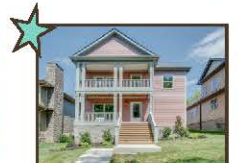
216 ORLANDO AVENUE Charlotte/White Bridge
